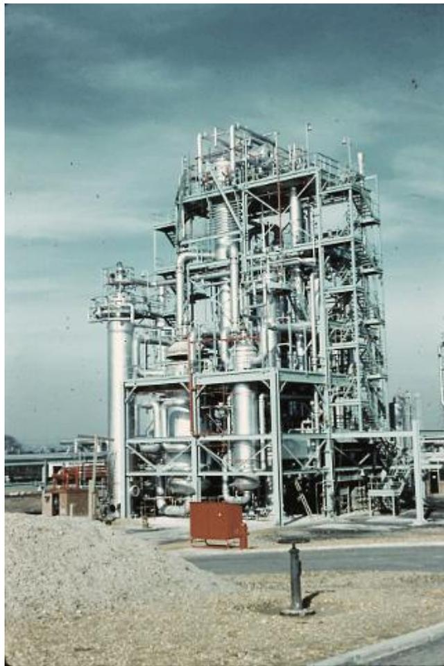
I inherited this picture, shows the finished the UCC Fawley Works in 1960-ish. It is an excellent technology photo, almost a portrait. The Southampton Water is in the background, where oil barges offload raw materials right into the continuous refining process at the Esso site, off to the right. This equipment is still visible (probably modified now) on Google Maps.
